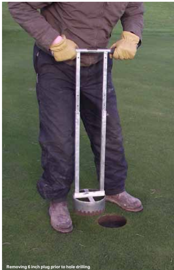
Removing 6 inch plug prior to hole drilling
