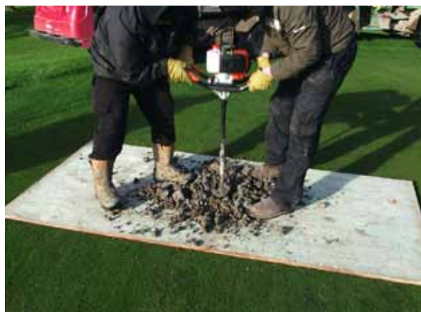
Drilling 1.3 metre hole with powered auger
