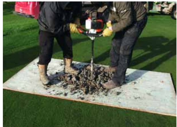
Drilling 1.3 metre hole with powered auger
