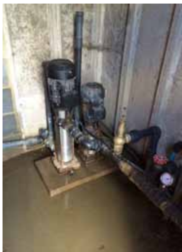
Example of a wet pump house floor
