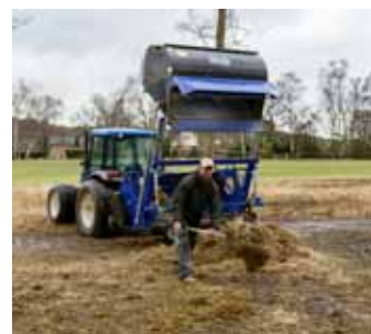
MAIN ABOVE: Ground cleared and surface prepared ready for heather brashings. INSET ABOVE: Spreading heather brashings over prepared area
