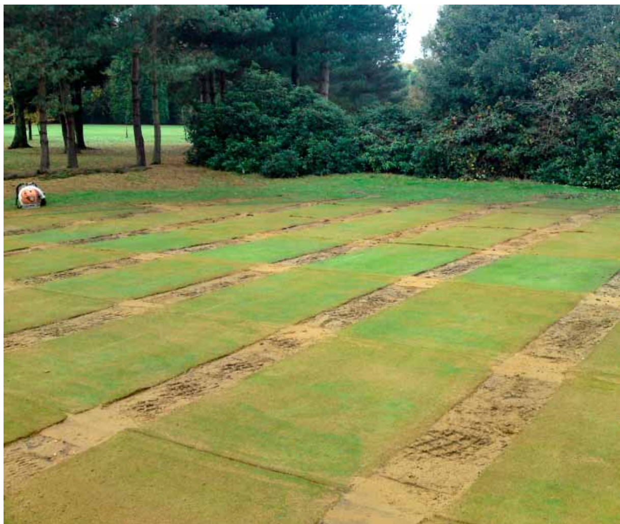
ABOVE: Greens drained via Wizz wheel trencher
