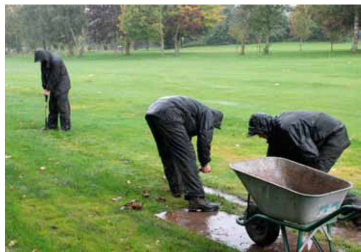
INSET ABOVE: Steve Castle digging in!
