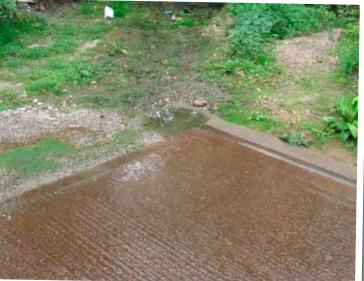
3. Machinery is washed down on a bunded washpad with all contaminated water fed by sealed pipe into a dedicated and bespoke reedbed system, where it is cleansed sufficiently for discharge or re-use.
