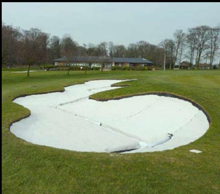
Bunker Solution is a three-part liner that answers many of the commonly occurring bunker problems. The three parts are the mat, anchor and drain liner. It provides "grip" for sand in the bottom bunkers and on bunker faces.
