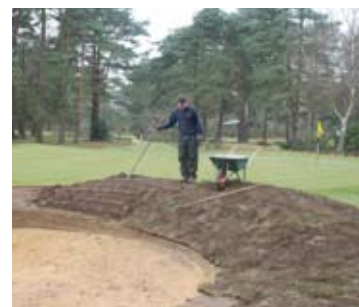
RIGHT and BELOW: part of the bunker renovation programme
