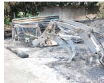
INSET ABOVE: More damage caused by the fire.
