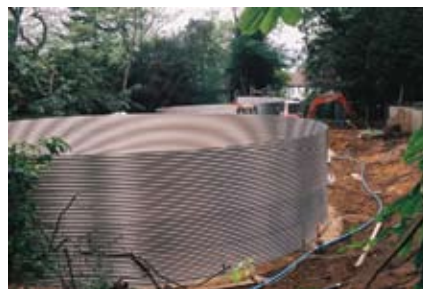
The water tanks at Tandridge under construction
