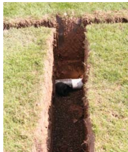
Trench at Northop GC - Copyright MJ Abbott Ltd
