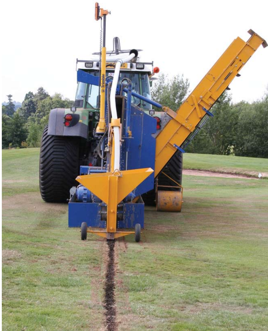
Trenching at Northop GC - Copyright MJ Abbott Ltd
