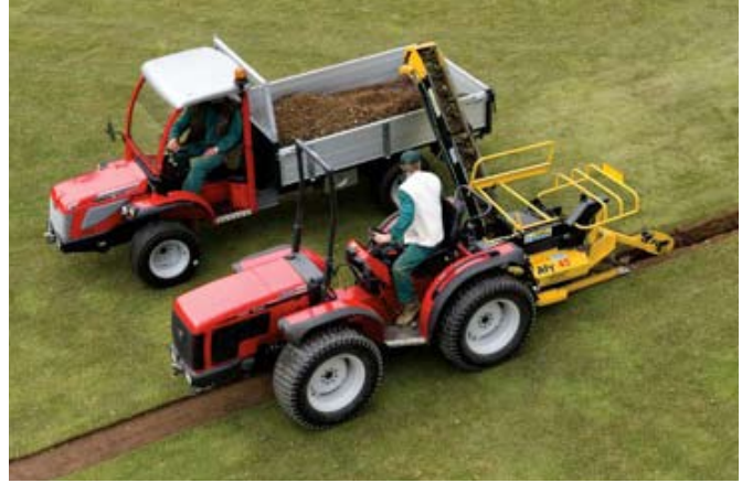
Trenching to install a pipe drain
