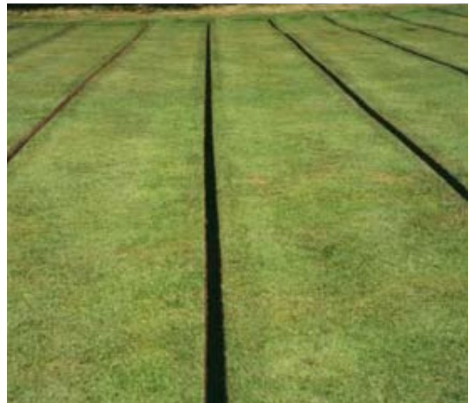
Neat clean trenching
