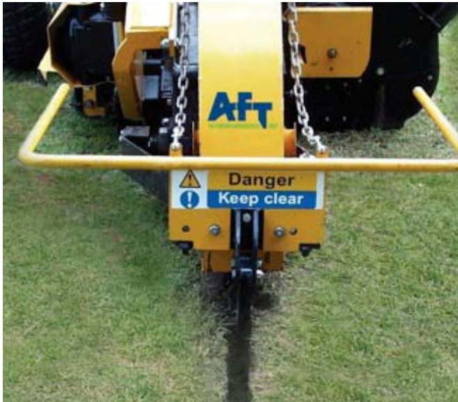
Narrow trenching for slit drains
