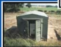
Irrigation Pump Housing
