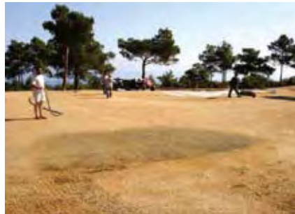
Picture 2: Spraying mulch mixed with water.
