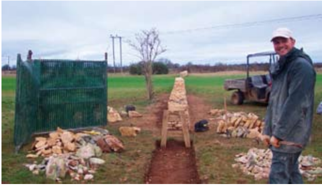
Large stones are put into the foundation and base courses, followed by progressively thinner stones for the uppermost courses.
