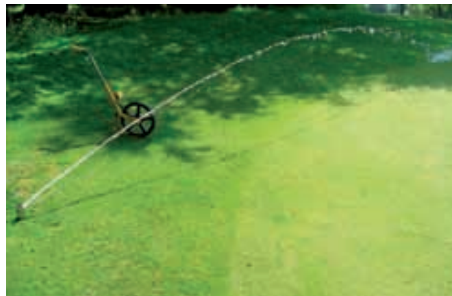
Poor pressure and droplet distribution
