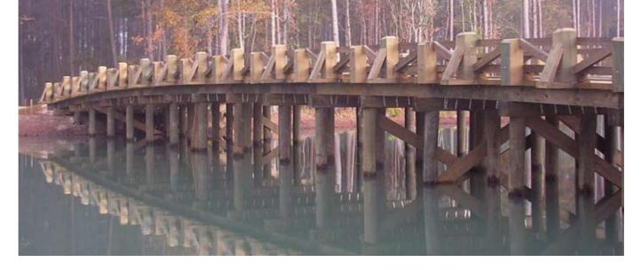
"If you want to reach 200 feet in a single span for example you are definitely looking at a steel bridge; from 10 to 20 feet you are looking at timber and for 30 feet a lot of people like to use a glue laminated beam timber," explained Richard, whose company, launched by Richard's brother Brian Nuttall, in 2000, is hoping to offer its services to UK customers in the near future.
