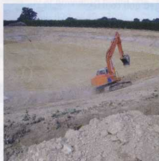
21 Building a reservoir
