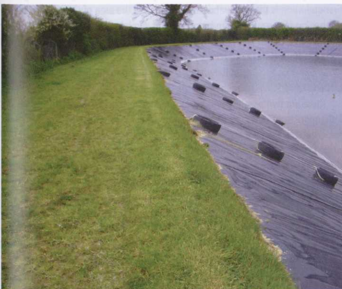
Finished embankment surface
