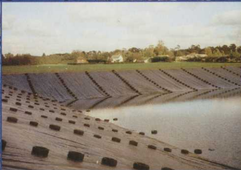
Frilford Golf Club: Irrigation Reservoir Liner
