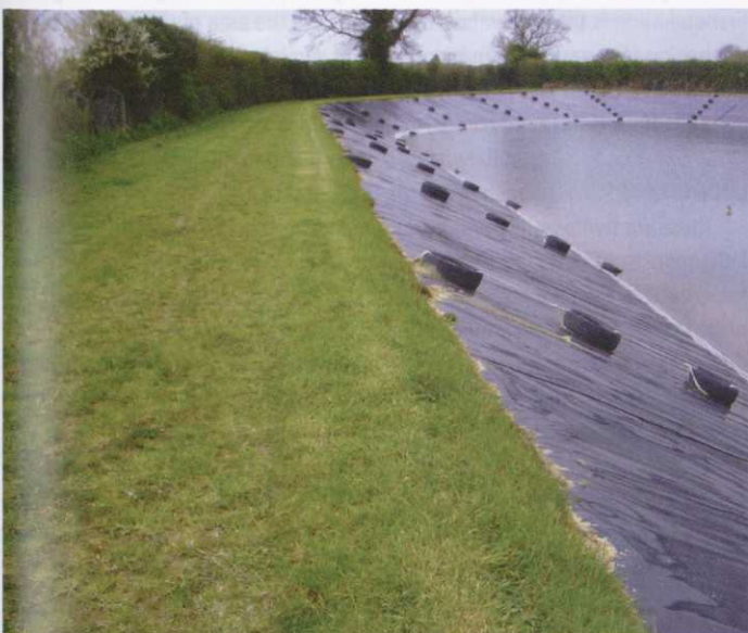
Finished embankment surface
