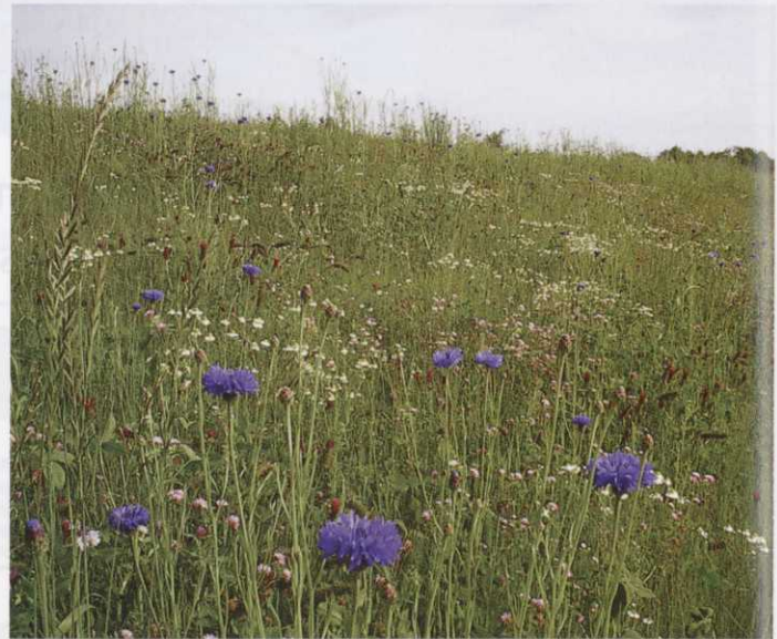
Synthetically lined reservoir embankment sown with a wildflower seed mix
