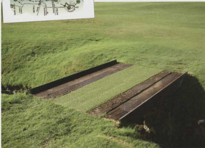
One of the recently built bridges
