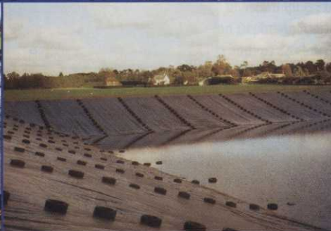
Frilford Golf Club: Irrigation Reservoir Liner
