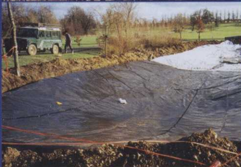
Donnington Grove Golf Club: Pond Liner
