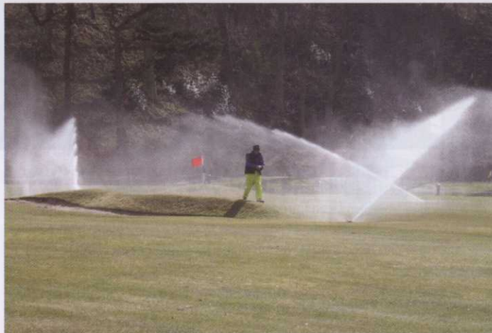
Overhead irrigation system operating on a golf green
