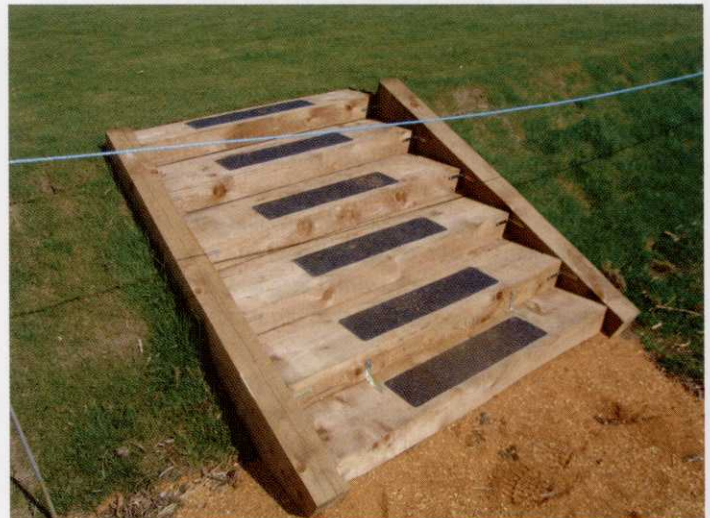
The team do all construction work in-house
