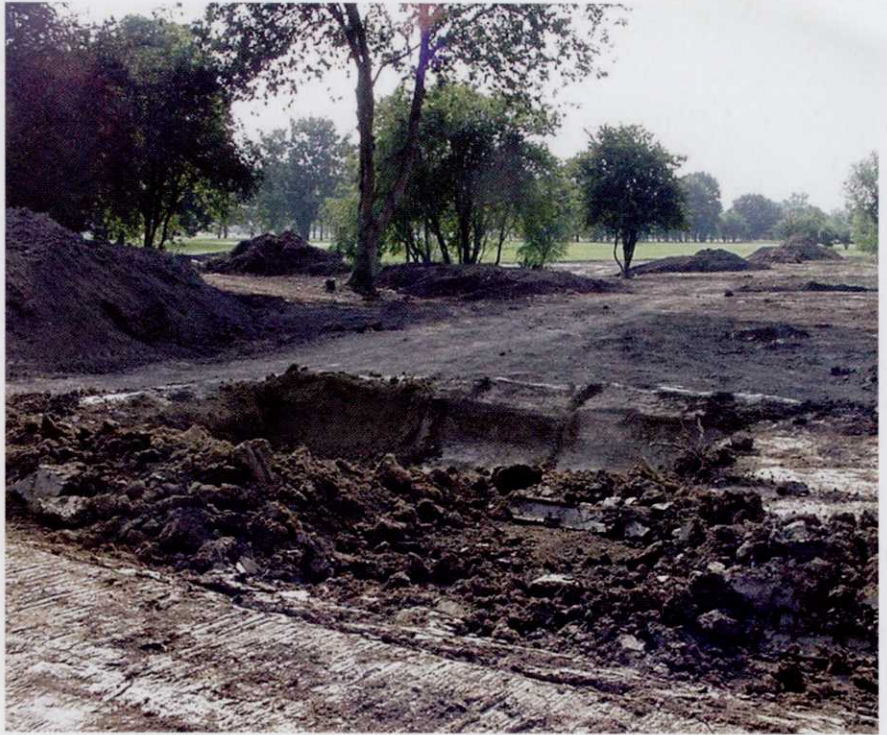
Preparation work for the new 13th green
