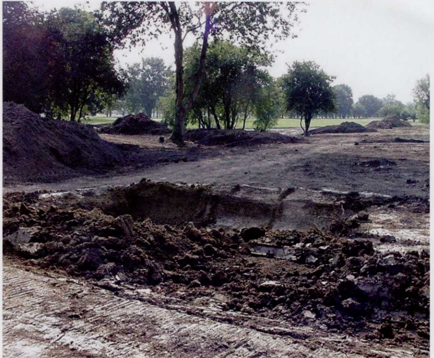
Preparation work for the new 13th green
