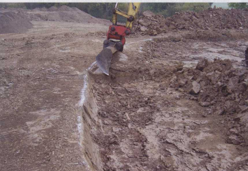
▲ Digging out the pit in ideal conditions
