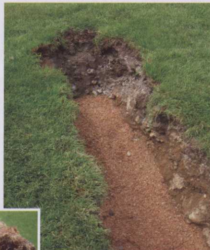
This ditch shows the quality of Loch Lomond's sub-structure
