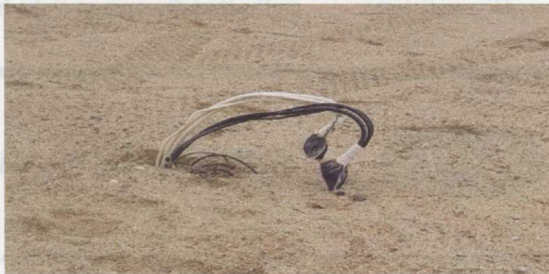
An example of good wire splices made using waterproof splice kits. Now they need to be placed in a valve box for protection and so they can be easily located later for troubleshooting if necessary
