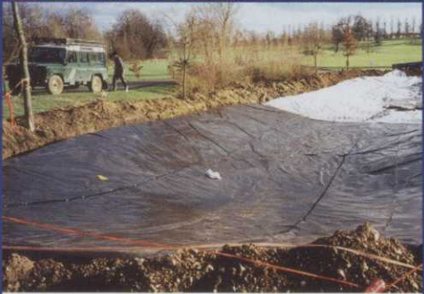
Donnington Grove Golf Club: Pond Liner
