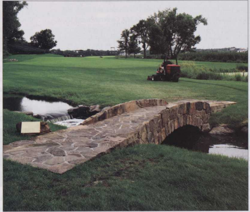
▲ A finely built stone bridge
