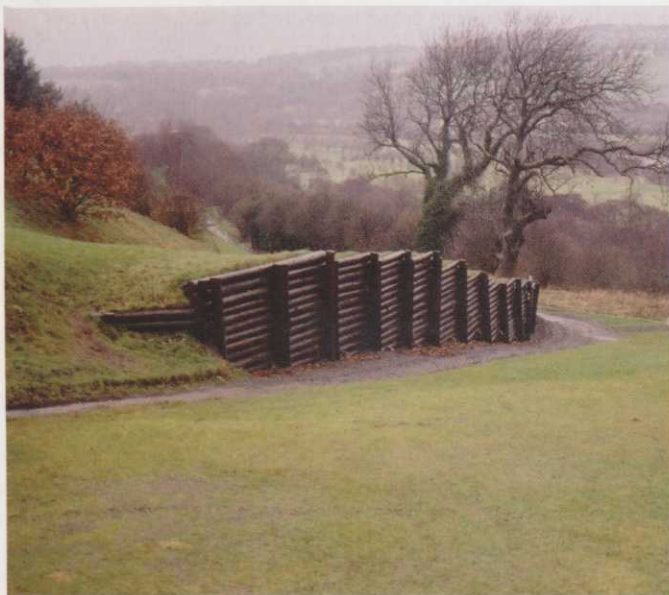
▲ The 14th hole with the public path shielded by the recently refurbished wall of sleepers
