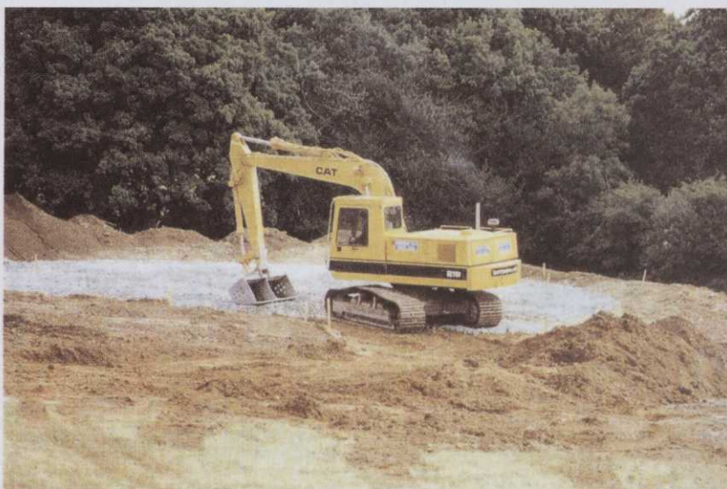
A blinding layer being spread by a long jibbed excavator.
