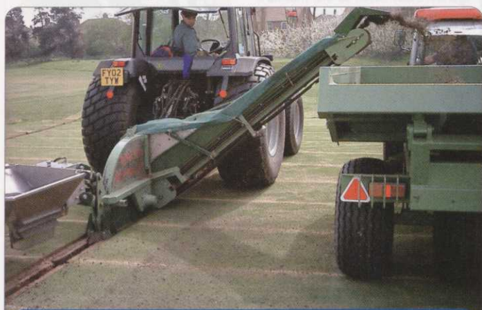
A trench being cut on a green prior to the installation of a 60mm pipe. Note the turf has been removed along the line of the drain. Bands running at 90 degrees to the pipe are 25mm trenches cut with a wheel trencher and filled with Lytag
