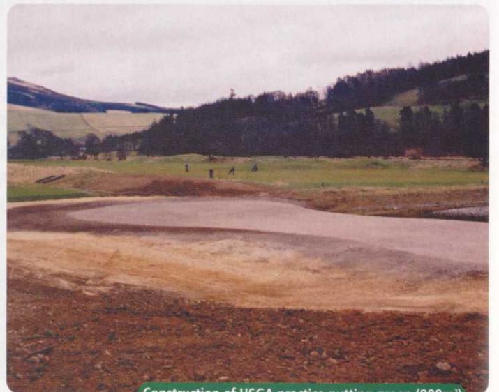
Construction of USGA practice putting green (800m 2 )
