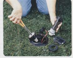
G870 has a 8.75 cm pop-up riser and a discharge rate from 50 to 120 liters per minute in a 14m to 23m radius. Color-coded, interchangeable nozzles are included.
