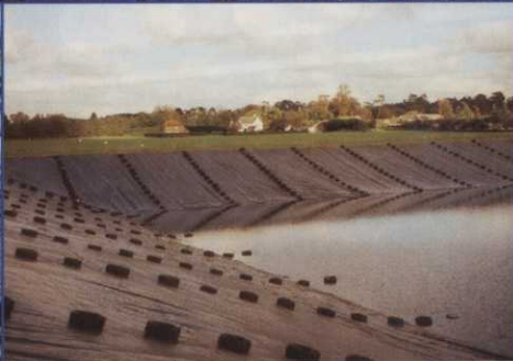
Frilford Golf Club: Irrigation Reservoir Liner
