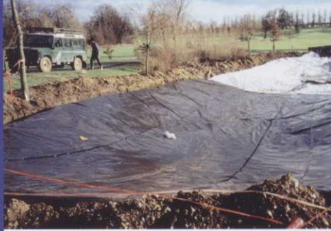
Donnington Grove Golf Club: Pond Liner
