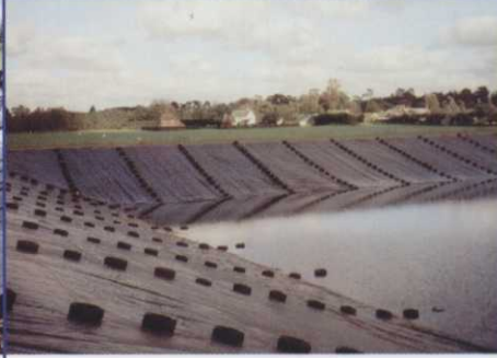
Frilford Golf Club: Irrigation Reservoir Liner
