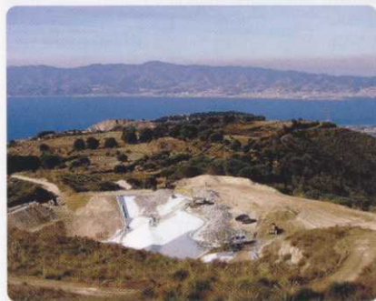
Photo 2: Installation of the lake shores
