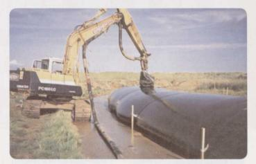
consultation with Maccaferri. Three geotubes were supplied to principal contractor J Breheny Contractors Ltd, each measuring 3.25 metres in diameter and 105 metres long. Filled with locally won sand, they form a solid core to the new coastal defences and will be able to withstand even severe winter storms. Maccaferri is the exclusive UK distributor for Geotubes, which are
