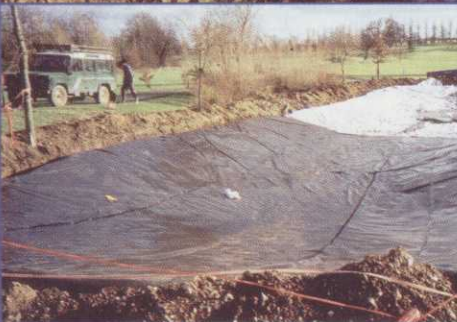
Donnington Grove Golf Club: Pond Liner
