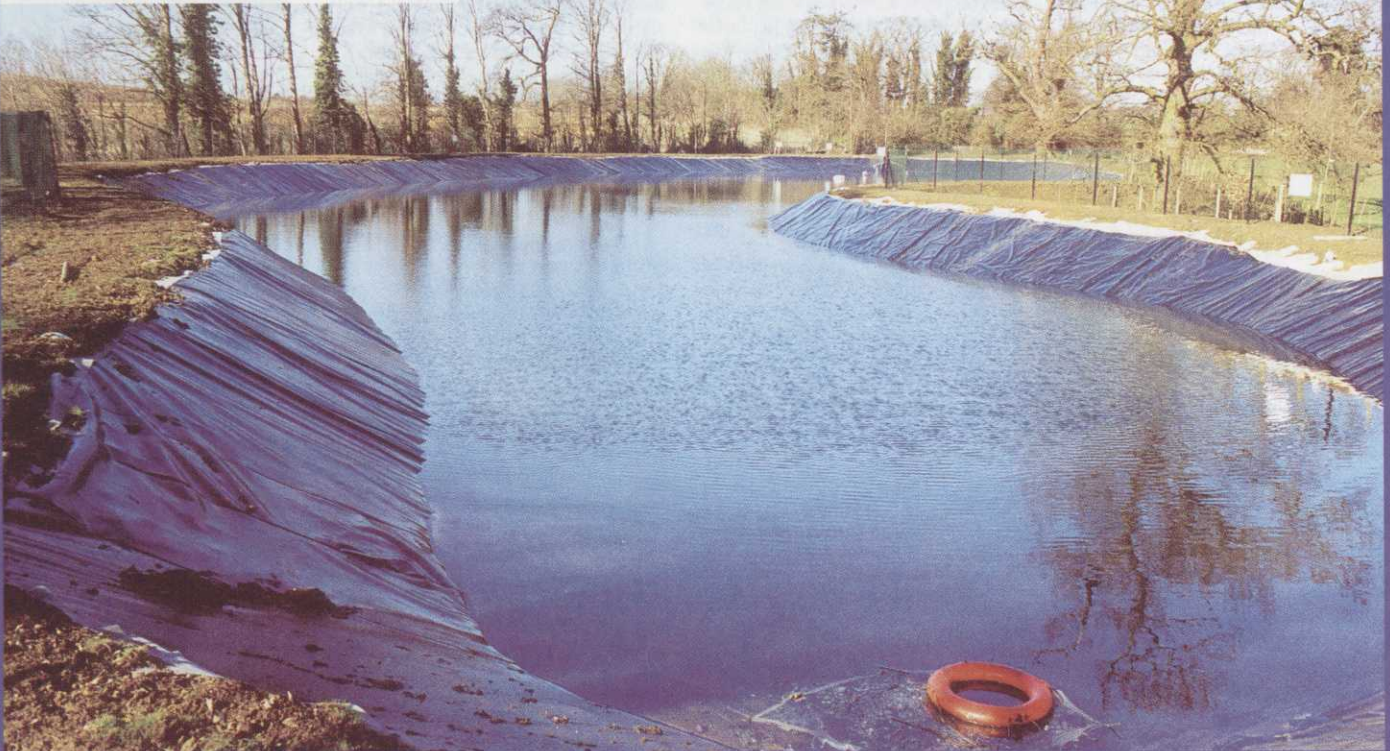
Hanbury Manor Golf Club: Reservoir Liner
