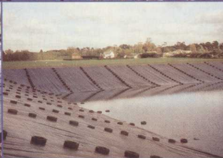
Frilford Golf Club: Irrigation Reservoir Liner
