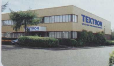
The Redditch branch has over 14,000 square feet of combined office, service and storage space.
