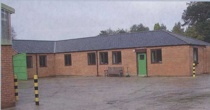
Below: The new maintenance facilities were designed to blend sympathetically to the surrounding buildings of Longdon Hall, and were fashioned on old stable blocks
