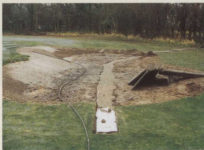
Far page: One of the new bunkers complete with steps
