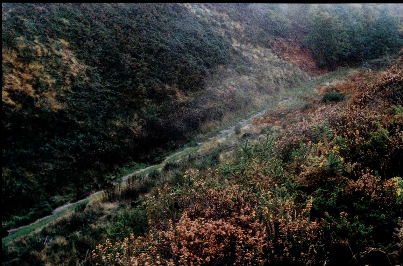
Above: The old railway cutting which runs through the course
