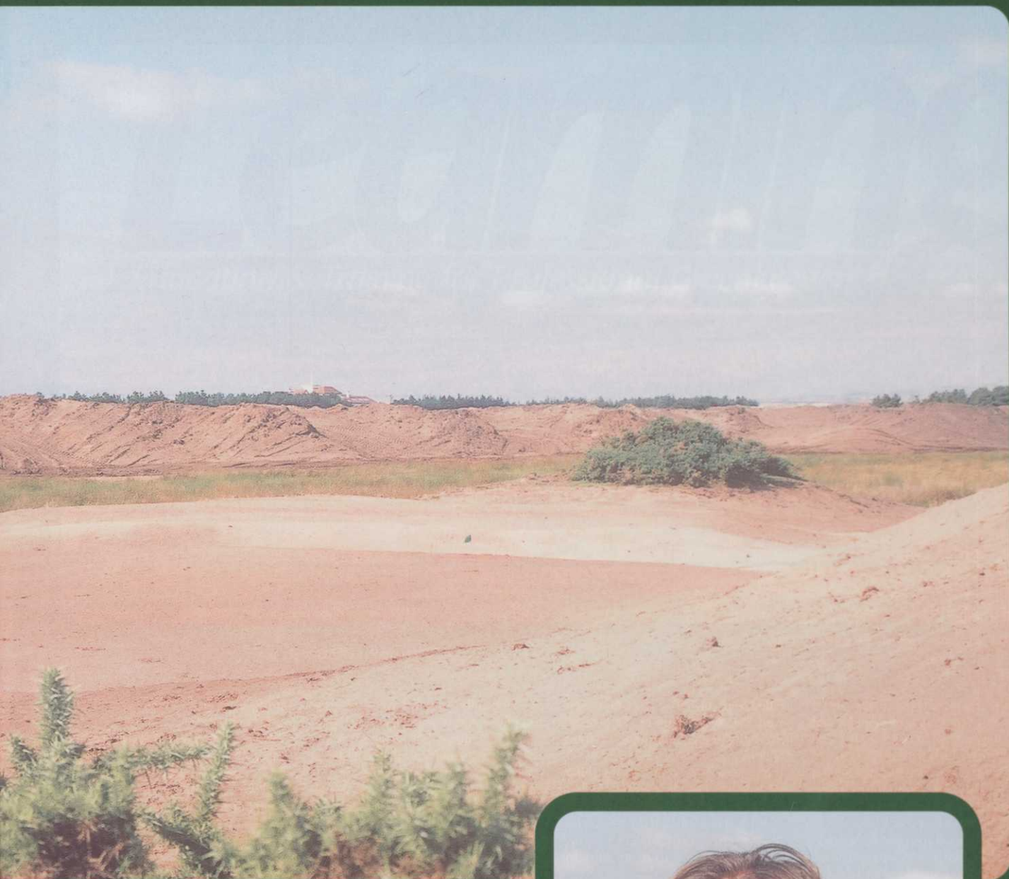
One of the distinctive Kyle Phillips greens under construction.
