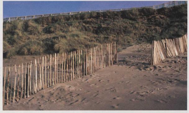
At Turnberry, fencing made from chestnut paling is staked into the top of a threatened dune to help prevent erosion
