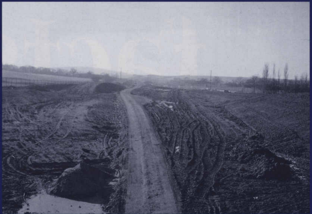
Right: Chesterfield Golf Course during the road construction
