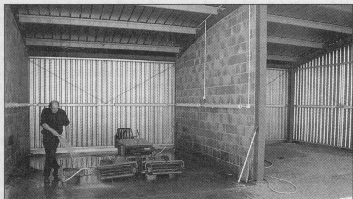
Separate wash bays are provided for cleaning course maintenance machinery
