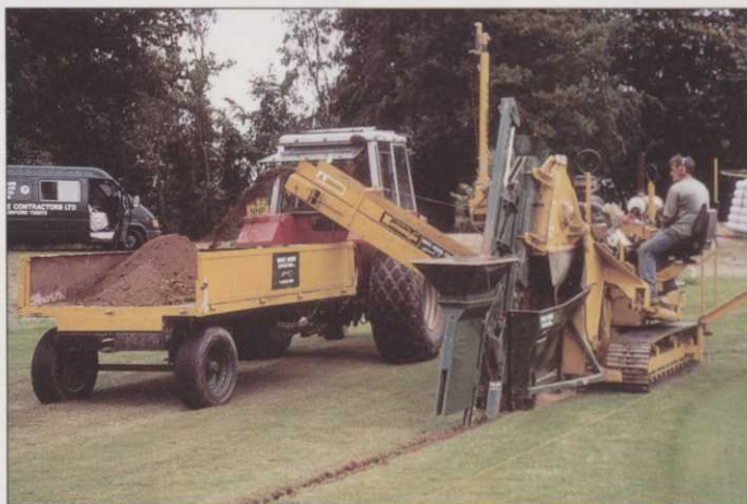
Drainage work in progress at Mill Ride Golf Club
